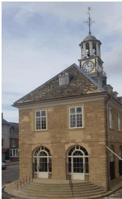
The entire building has been restored, with new stonework replacing those blocks that had suffered from decay, some 60% of the roof tiles replaced, the clock cleaned and serviced, and a new bell installed (from Taylors Bell Foundry in Loughborough).
